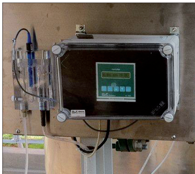
Typical installation example with controller CL 7685 and flowcell SZ 7231
